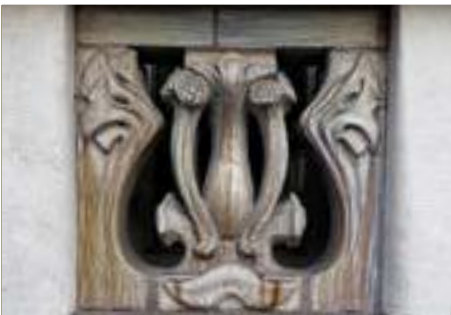
Laviurette Building, Paris
