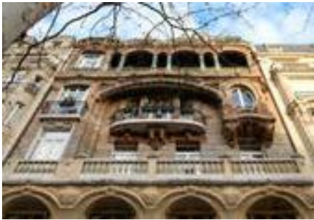
Laviurette Building, Paris
